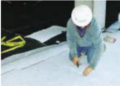
Preparing to complete installation of Enkamat 7918R over Enkasonic.
